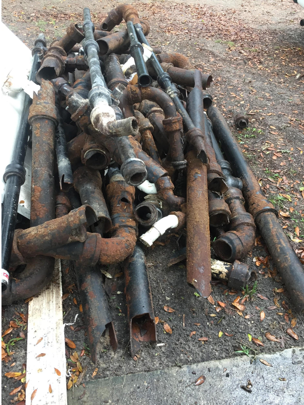
A pile of old waste lines
