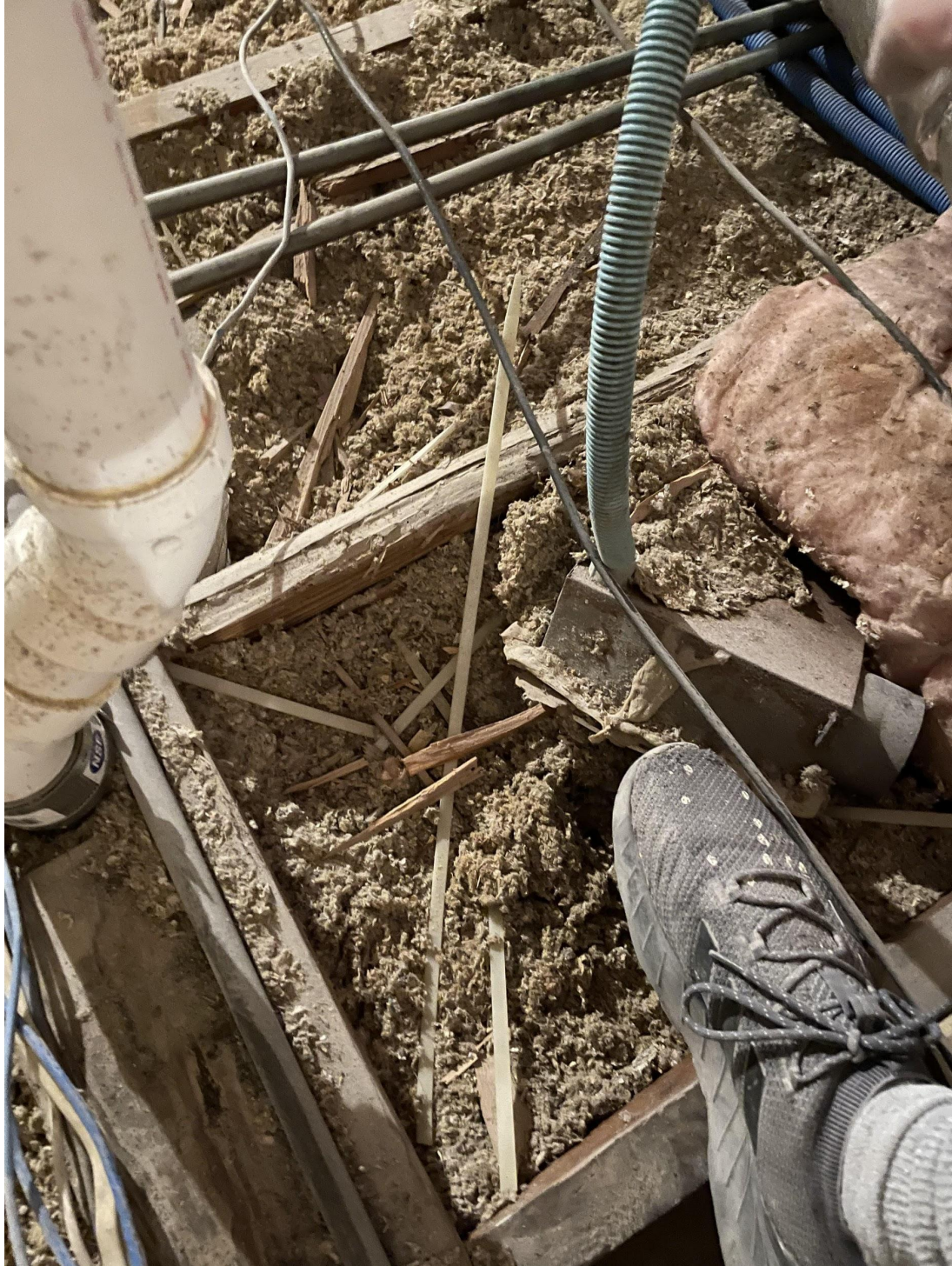
bathroom fan buried in insulation still wired live
