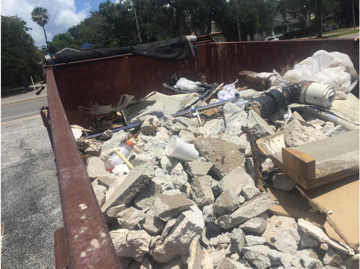
One of many trailers filled with concrete and debris
