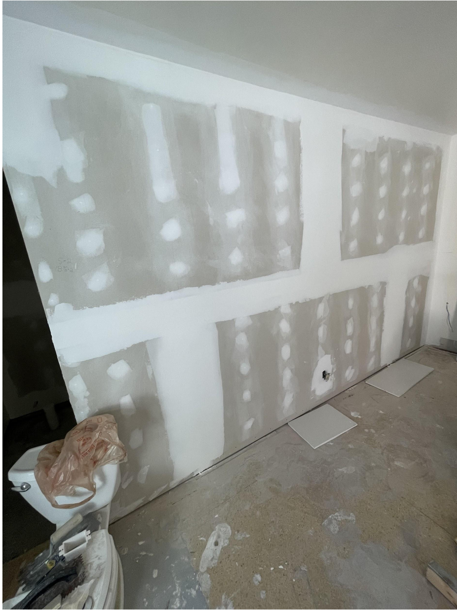
New drywall up in room 12
