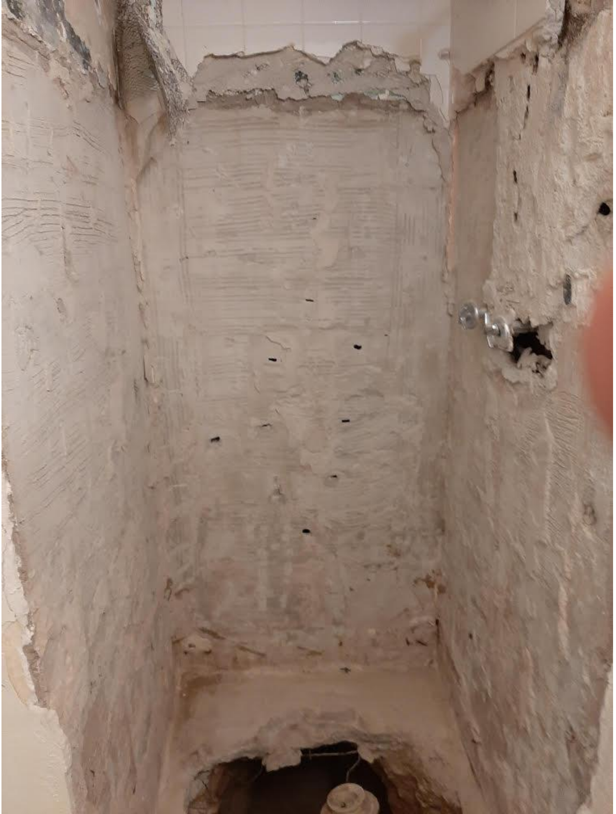
Chiseling out an old shower
